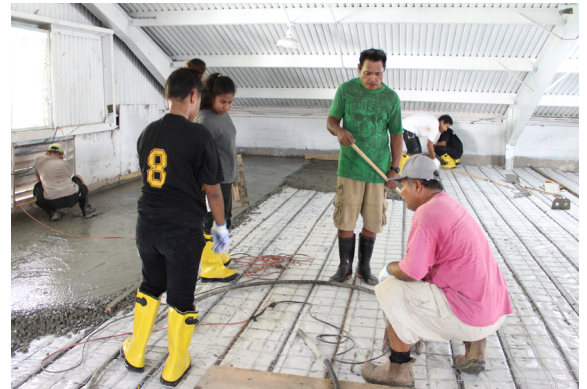
CTE Lab School students with Director of Physical Plant Clement Kazuma during concrete pouring at Temekai Bldg.
