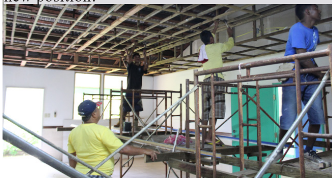
On October 22, 2019 PCC Conference room ceiling being replaced
