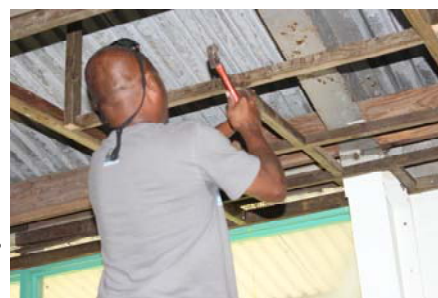
Installation of new LRC ceiling
