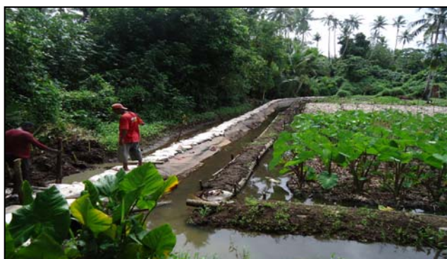
Dikes built to secure salt water intrusion from Mangrove
