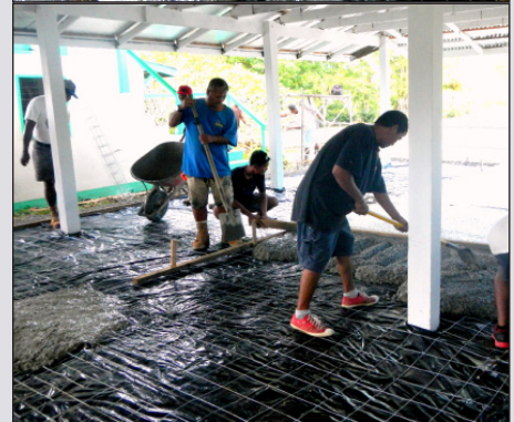
PCC Maintenance Workers building a new hut on the school campus.
