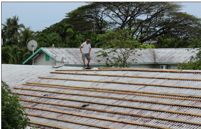
Maintenance workers repairing and re-roofing the Learning Resource Center (LRC) Office.
