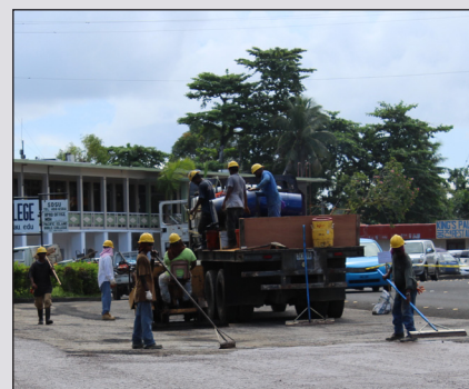
Workers applying a new layer of asphalt to the PCC main parking lot.
