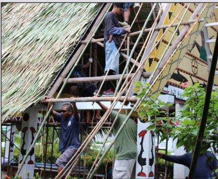
Workers re-thatching the roof of the bai.
