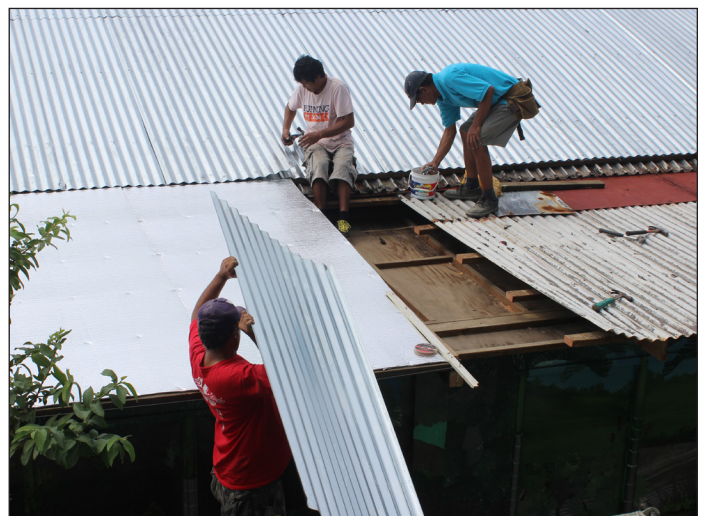
Workers roofing and repairing the college buildings with newer materials while adding insulation.
