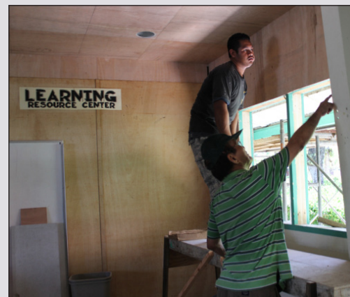
PCC maintenance workers working to renovate and improve the LRC facility
