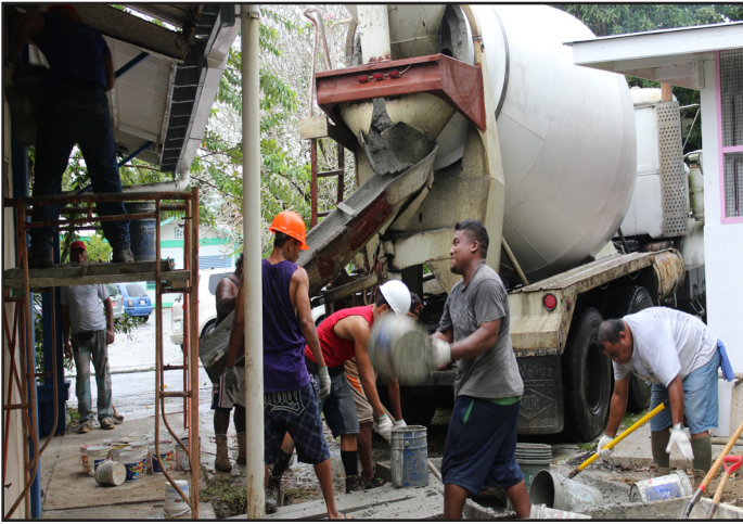
PCC maintenance staff and Construction Technology students during concrete pouring phase of the renovation.
