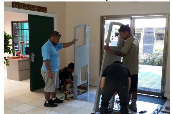
PCC Maintenance and library personnel participate in the installation
