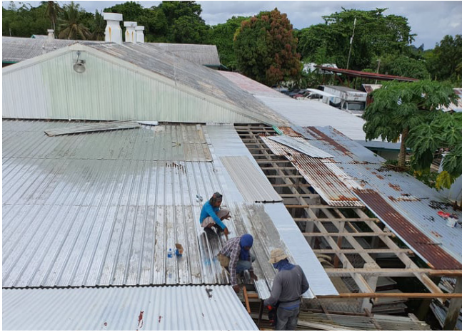
SEOM classroom & laboratory roof replacement
