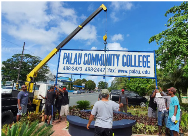
Utilizing crane truck to finally raised PCC signage
