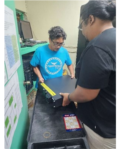
Installing backup batteries for servers
