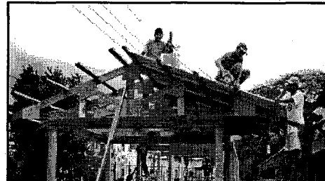
Maintenance guys laying the tin roofing for first hut.
