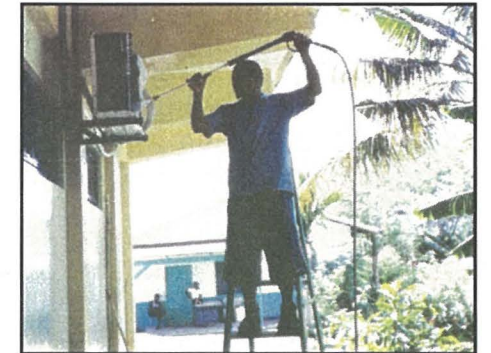
Student Clentin Saeuilil cleans air condition unit with water blaster
