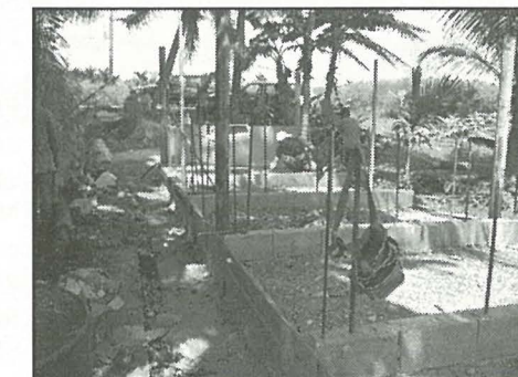
Dry Litter System still under construction at John Oiph's farm.
