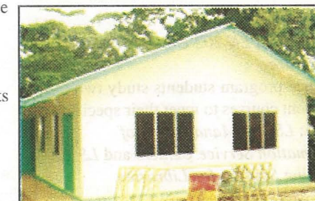
New Construction Technology building that will house architectural drafting classes and office.
