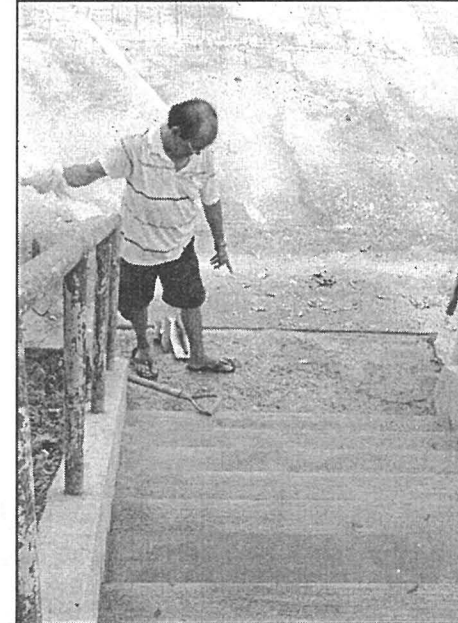
Rogelio Vergara inspecting the cement stairs he just repaired.
