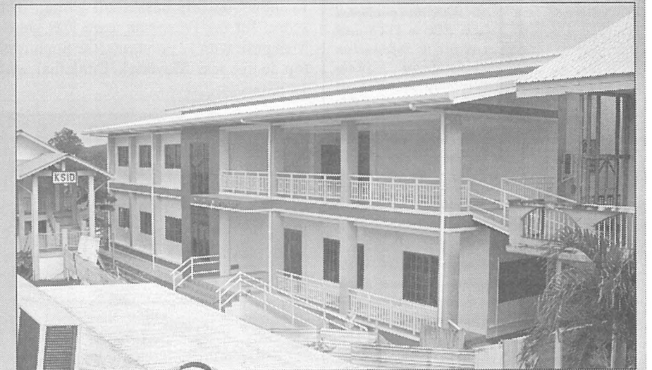
The air conditioners are whirring and final walkthroughs are being conducted. That is one nice library. The newly constructed building will house the library collections on the first two floors while the top floor will be used for faculty offices and the ASPCC office.
