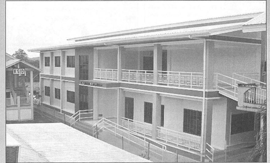
It's done! Last week we conducted final walkthroughs and we will soon begin transferring books and other materials into the new building. The newly constructed building will house the library collections on the first two floors while the top floor will be used for faculty offices and the ASPCC office.
