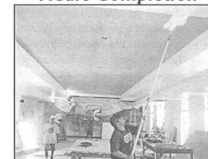
Maintenance crew paint the roof of the new assembly hall.
