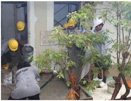
CTE STUDENTS & PCC STAFF AT TEMEKAI BLDG.
